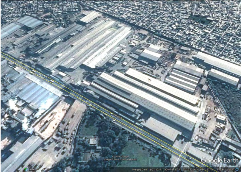
A Google Earth view of the Isgec Plant at Yamunanagar (Haryana), India
