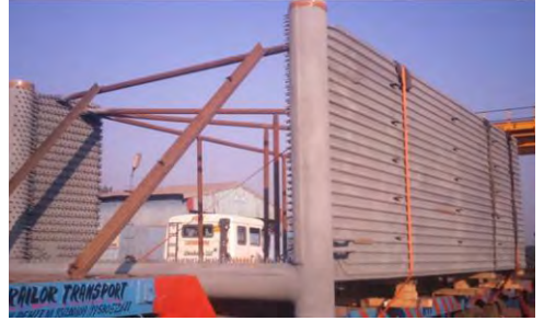
CFBC, Semi Assembly Cross Over Duct
