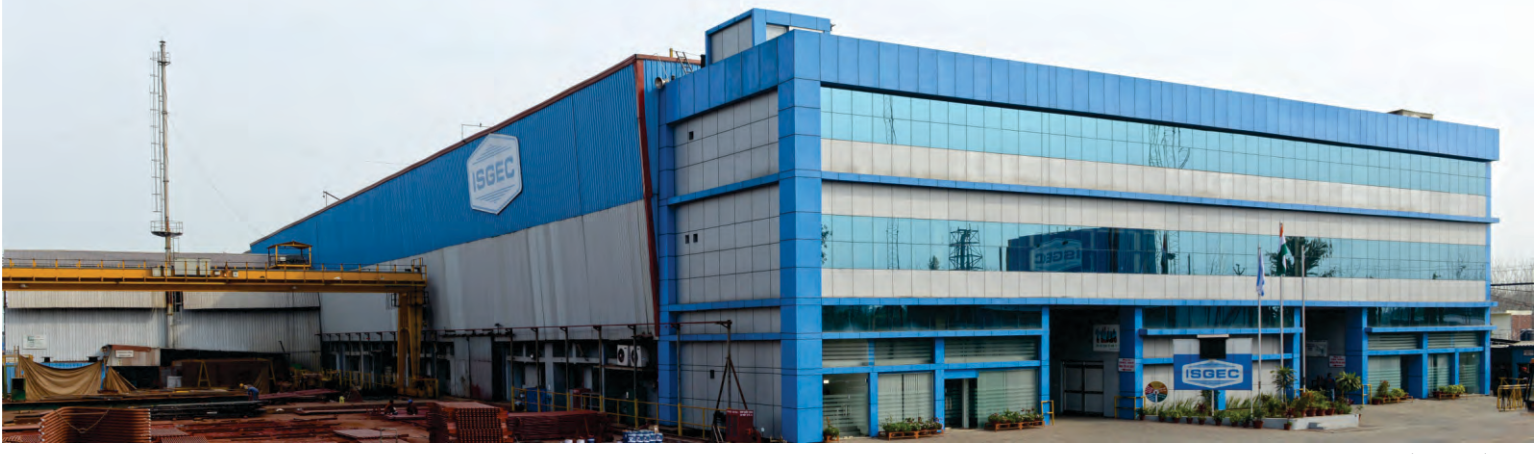
Boiler Pressure Parts Plant at Rattangarh (Haryana) India The Plant has a covered Shop Area of 16,650 sq.m. We also have additional adjoining land area for quick & easy expansion
