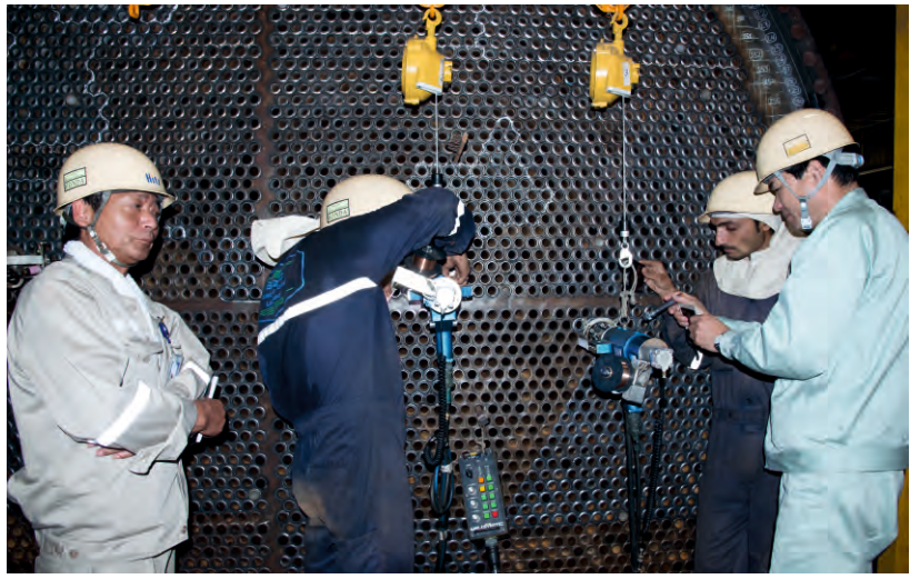
Automatic Tube to Tube Sheet Welding in EO Reactor
